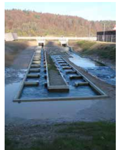
Ribja steza ob hidroelektrarni Blanca na reki Savi Fishway at the hydro power plant Blanca on the Sava river
